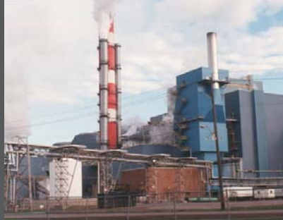
Temporary Smoke Stacks
